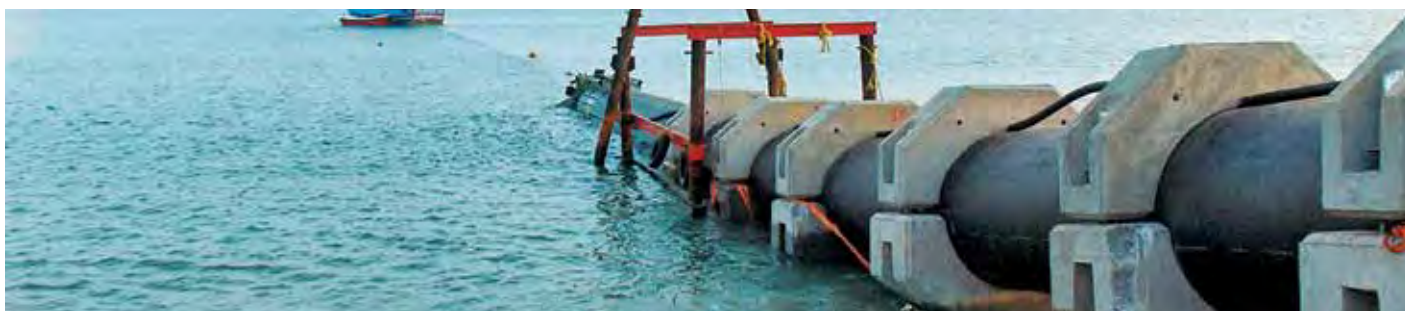
A view of the pipe line (1600 mm) used in the desalination project at Chennai (2008)
